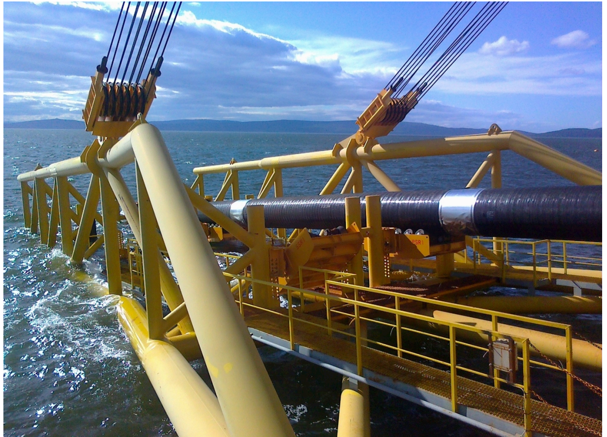
Laying gas pipelines through Nevelsky Strait
