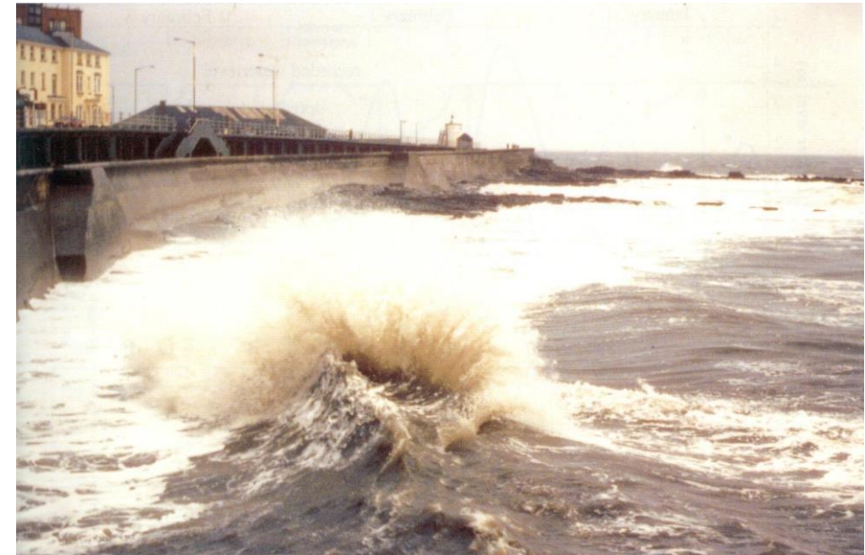
Reflection in front of the seawall at Port Cawl, UK
