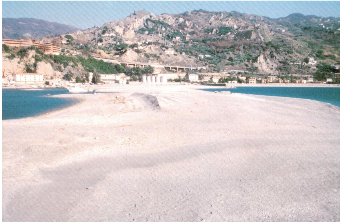
Complete siltation of a harbour entrance, Calabria, Italy
