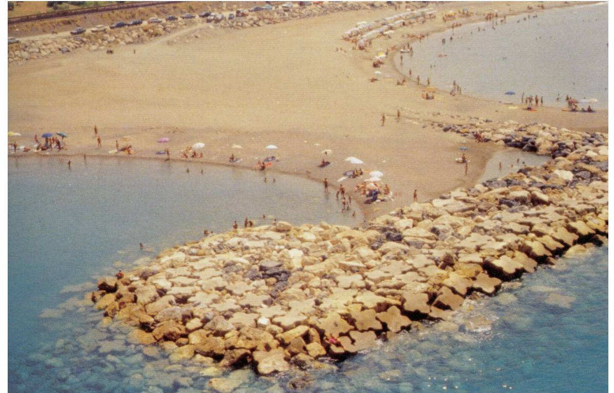
A T-shaped breakwater armoured with concrete units, a tombolo has formed behind it, Calabria, Italy
