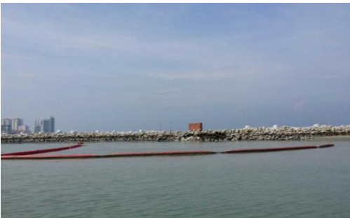
(a) Installation of silt curtains in front of a discharge outlet
