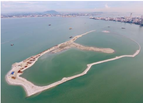
Fig. 18. Sand feeding at the artificial island enclosed by perimeter bunds by a TSHD [4].
