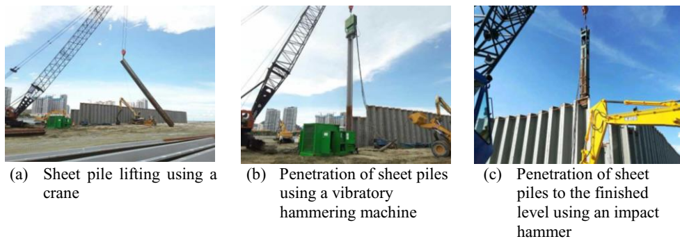
Fig. 27. Sheet pile installation.
