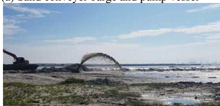
(c) Pumping sand through a discharge pipe from a dredger
