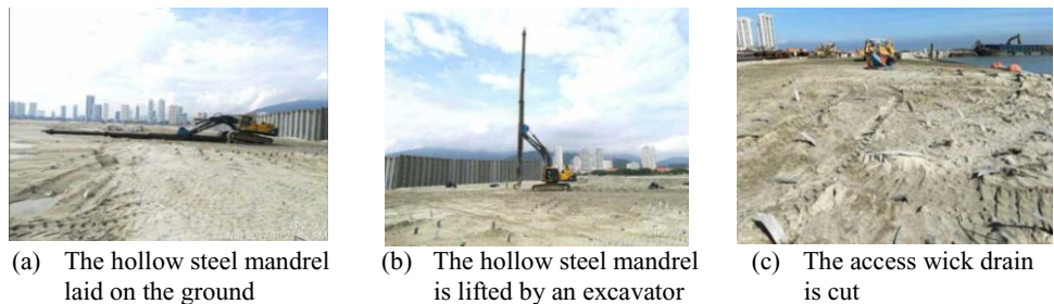
Fig. 23. PVD installation at the STP2 sand island.
