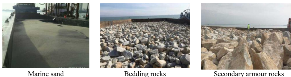
Fig. 15. Delivery of construction materials using barges.
