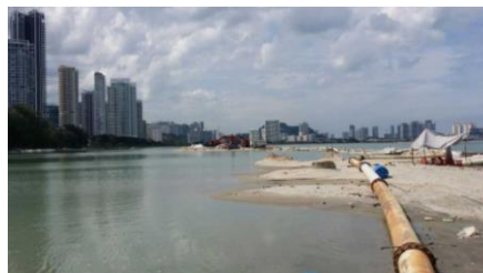
(b) Delivery of sand via pipeline
