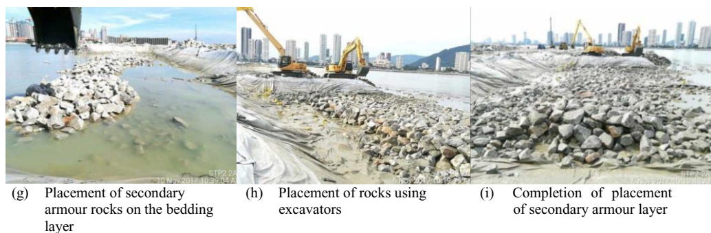
Fig. 29. Construction sequence of revetment
