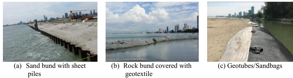
Fig. 7. Perimeter protection used for the STP2 reclamation.
